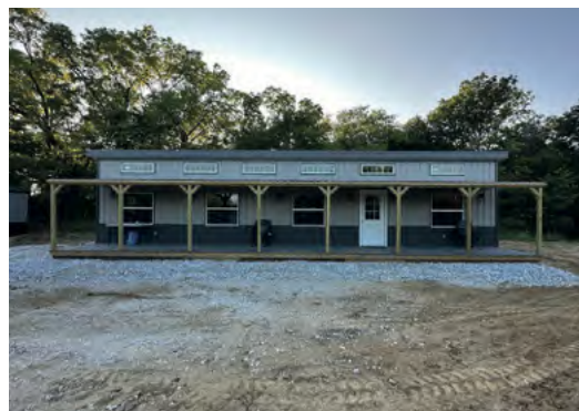
14'x44' Navy & White Paint (LP® SmartSide®); Black Metal Roof. (Shown with insulated windows.)
