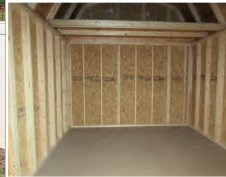
12'x12' Lofted Barn – Light Gray & Dark Gray Paint (LP® SmartSide®); Charcoal Metal Roof
